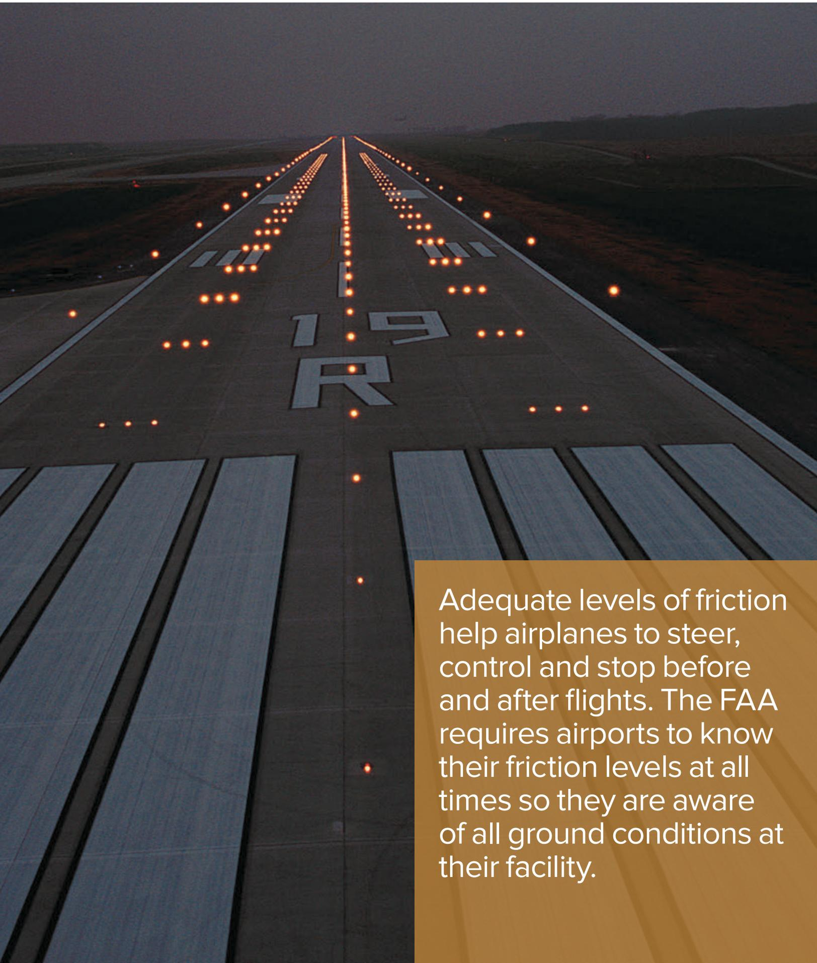
Adequate levels of friction help airplanes to steer, control and stop before and after flights. The FAA requires airports to know their friction levels at all times so they are aware of all ground conditions at their facility.
